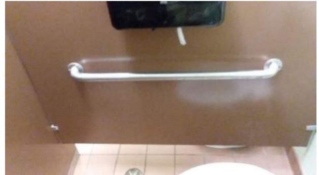
Missing Vertical Grab Bar
