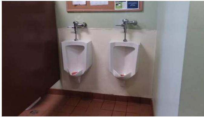
One Urinal Required to be Accessible when More Than One is Provided
