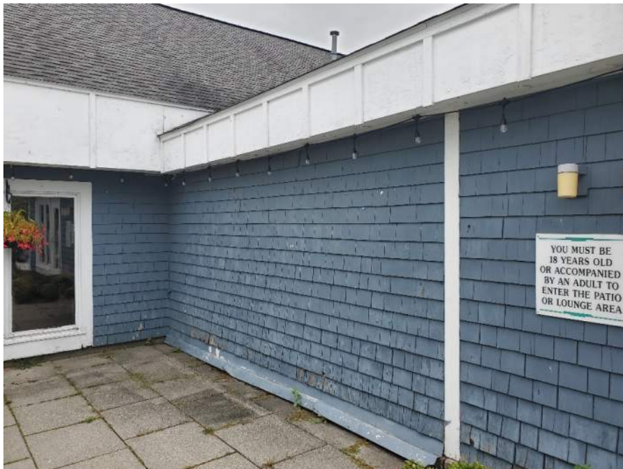
Damaged Siding & Roof Fascia
