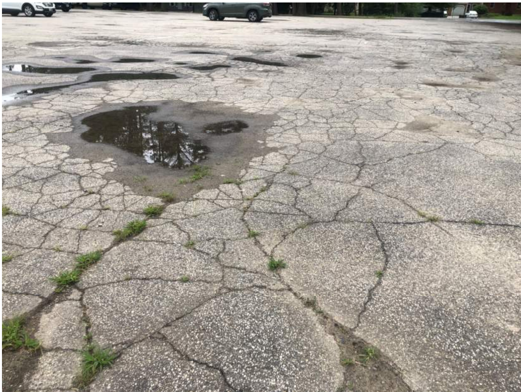
Badly Cracked and Deteriorated Pavement - Typical for All Areas of Parking Lot
