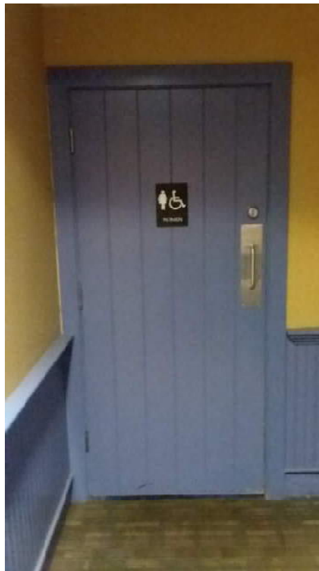
Accessible Restroom Signage Required on Wall Adjacent to Pull Side of Doors – Not Mounted on Doors
