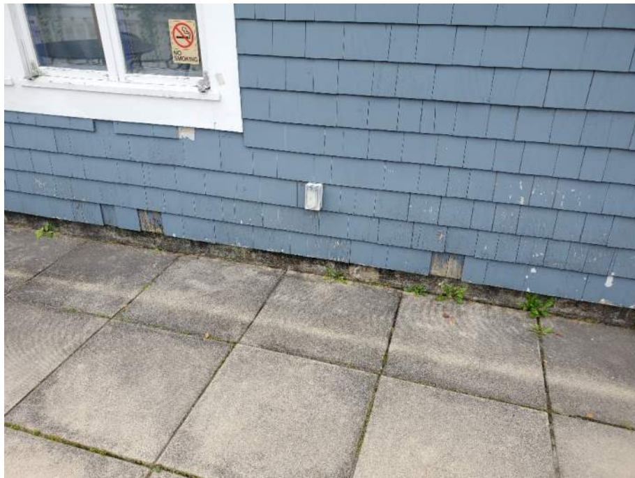
Damaged Siding on North Side
