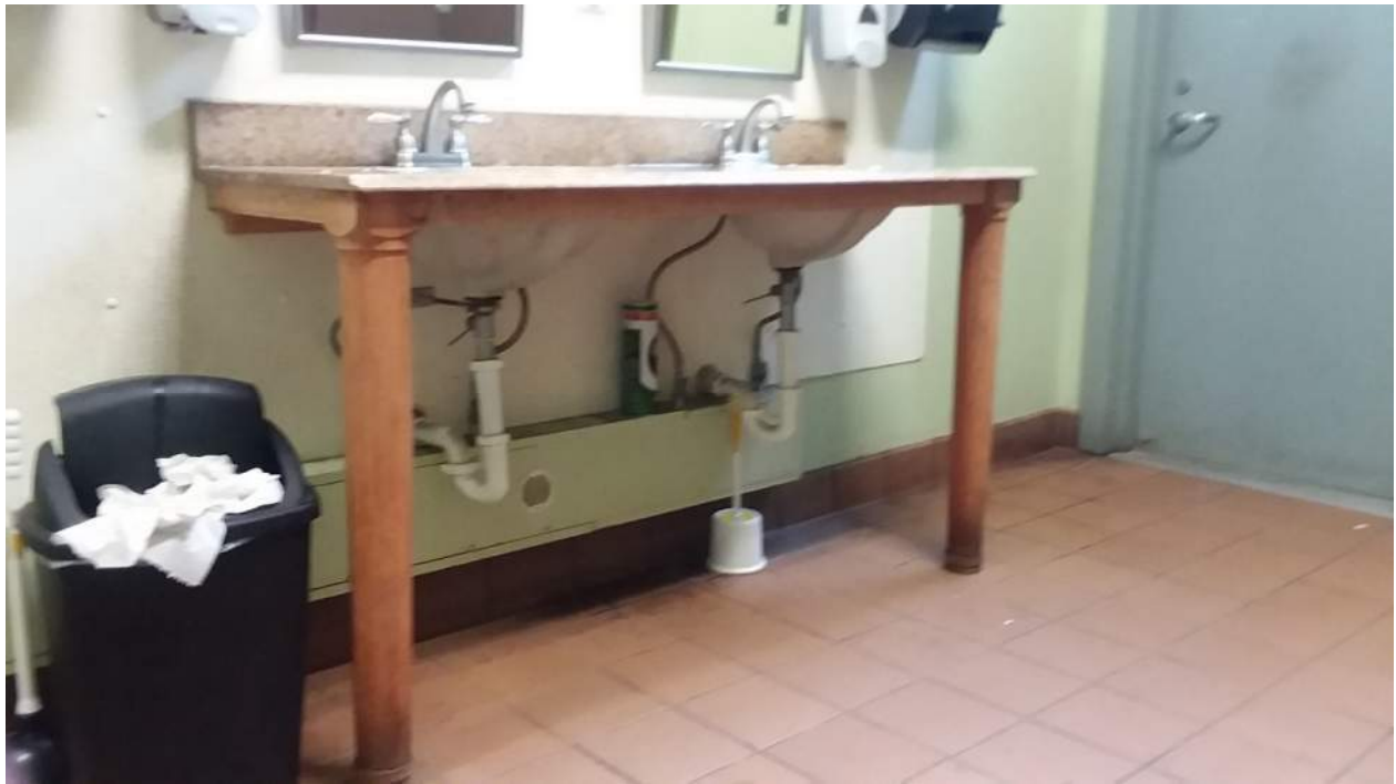
Plumbing Pipes Unprotected from Contact by Persons in Wheelchairs
