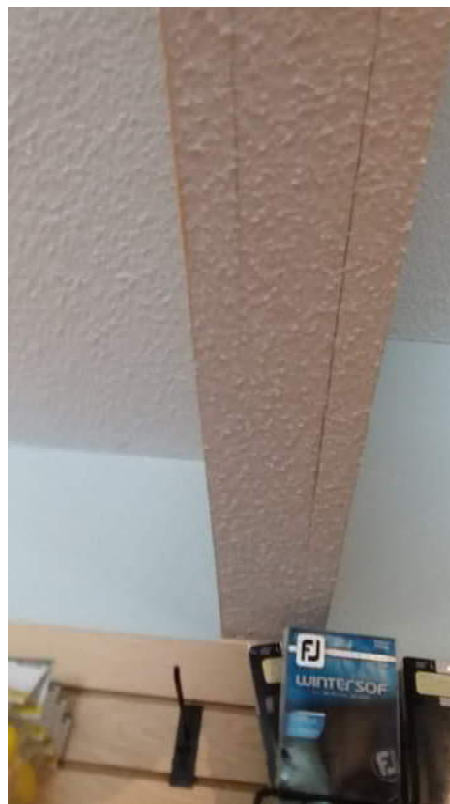
Beam Cladding Finish in Pro Shop
