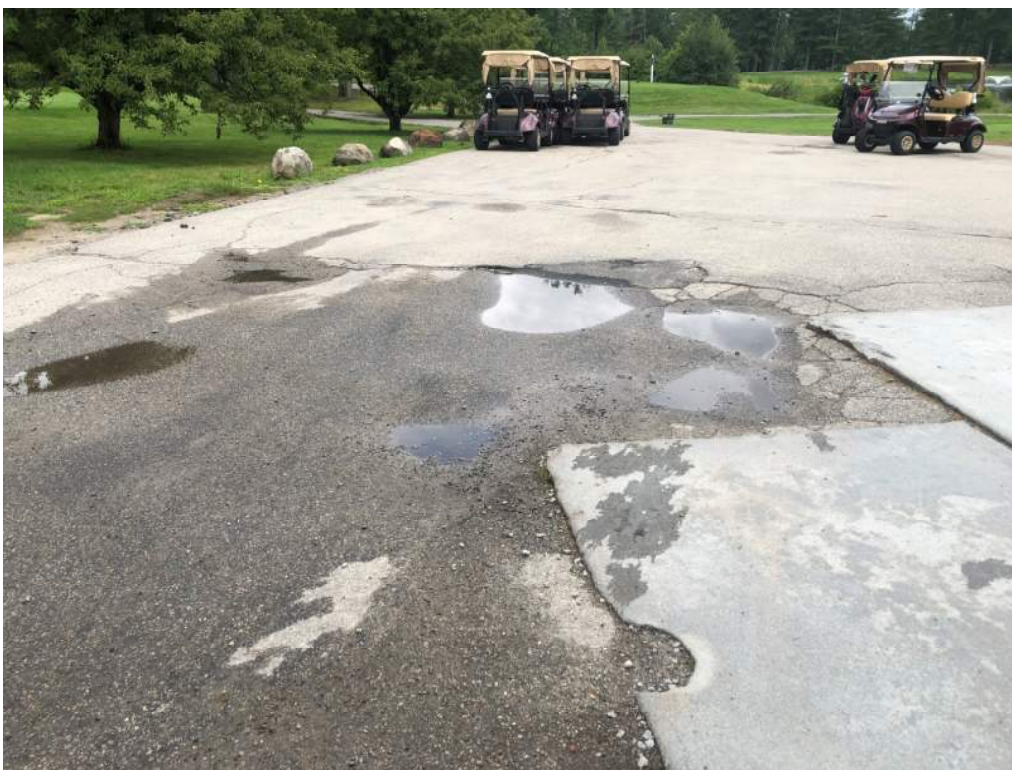
Ponding, Cracked Pavement, Collapsed Edges, Broken Hardscaping, Tripping Hazard – Northeast of Club House
