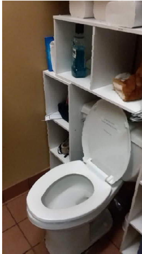
Compliant Smooth, Hard, Nonabsorbent Wall Surfaces Required within Two-Feet of Toilets & Service Sinks
