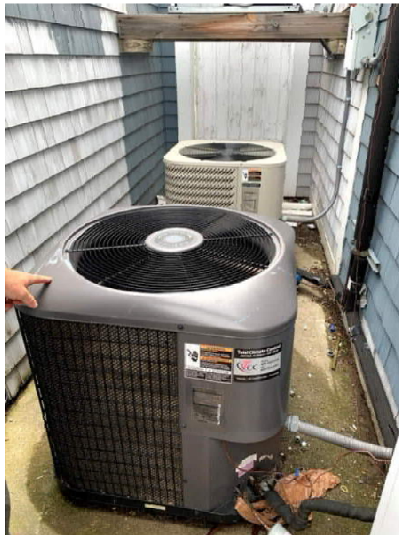
Air conditioning condensing units
