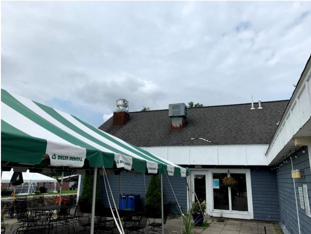
Intake and exhaust fan for kitchen hood
