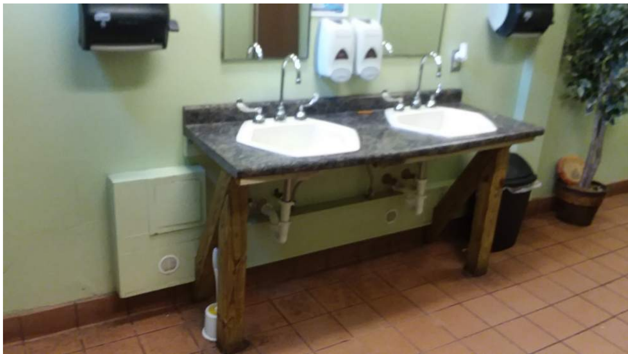
Plumbing Pipes Unprotected from Contact by Persons in Wheelchairs
