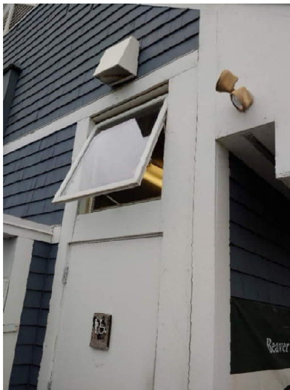
Incorrect Signs on Inaccessible Restroom Entrance
