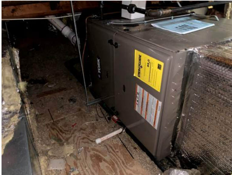
Function Room 5 ton air handling unit
