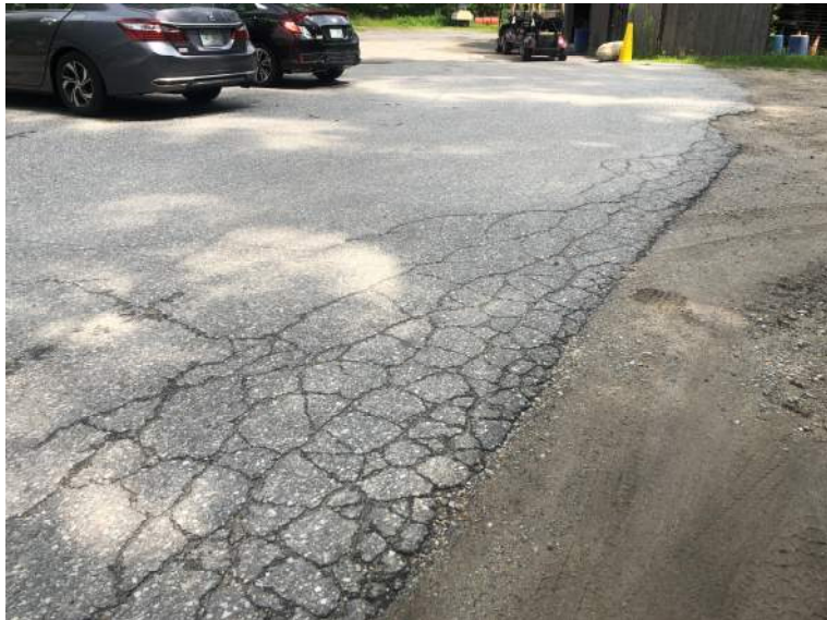
Typical Collapsed Edge of Bituminous Pavement Around Perimeter of Most Paved Areas
